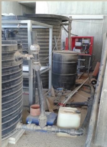
Candidate system (Membrane Bioreactor) for both Abu Dis and HUIJ/Givat Ram campus
