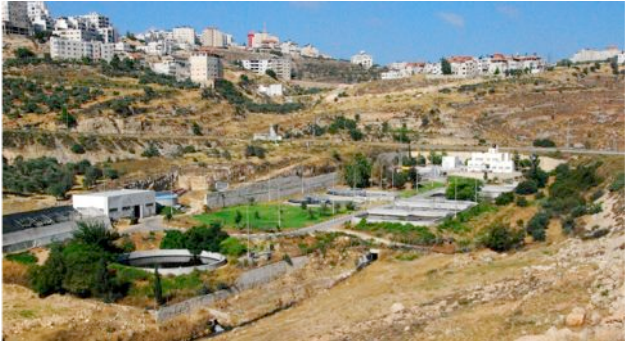
One of few large-scale wastewater treatment plants in the Palestinian West Bank (photo credit: Moses Jackson)
