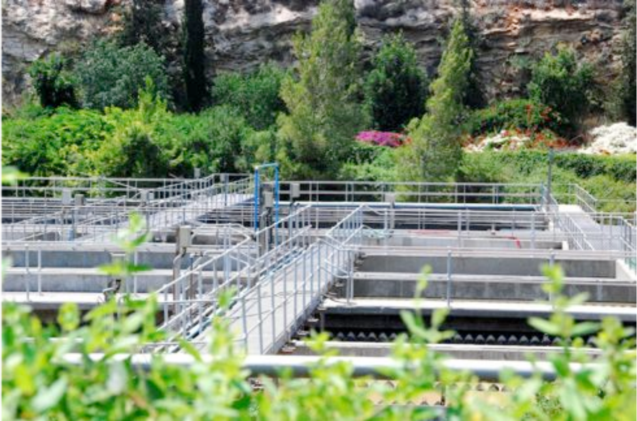
Aeration tanks at the Israeli wastewater treatment plant in Soreq (photo credit: Moses Jackson)
