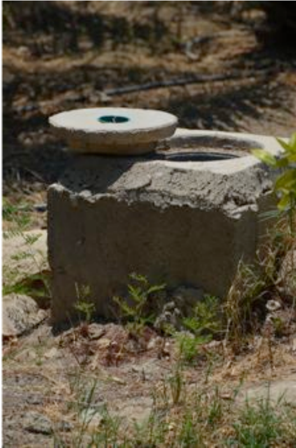
Onsite graywater treatment infrastructure in Al 'Oja (photo credit: Courtney Owen)
