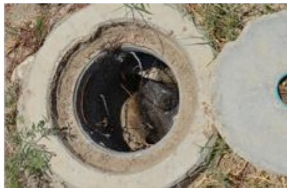
Onsite graywater treatment infrastructure in Al 'Oja (photo credit: Courtney Owen)
