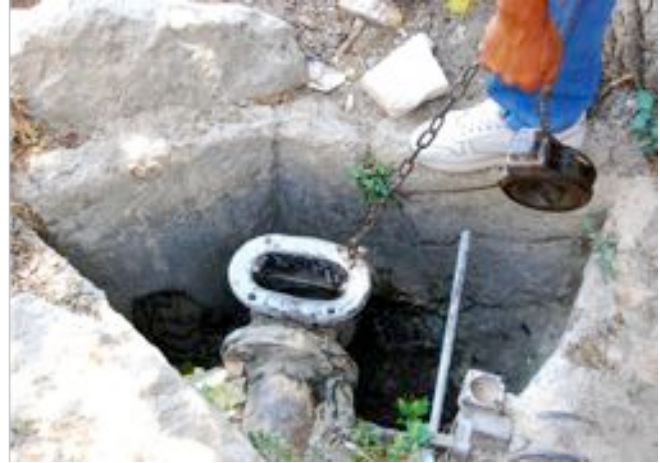
Sluice gate used to divert agricultural water in Battir (photo credit: Moses Jackson)
