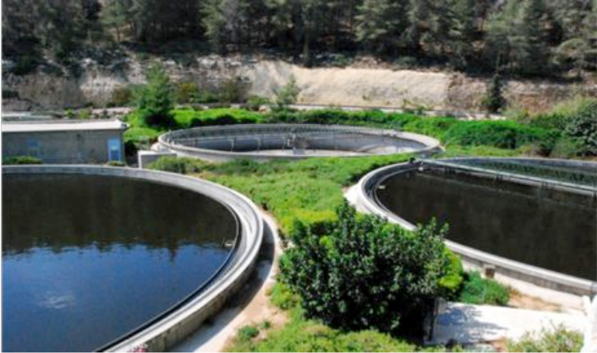
Settling tanks at the Israeli wastewater treatment facility in Soreq (photo credit: Moses Jackson)
